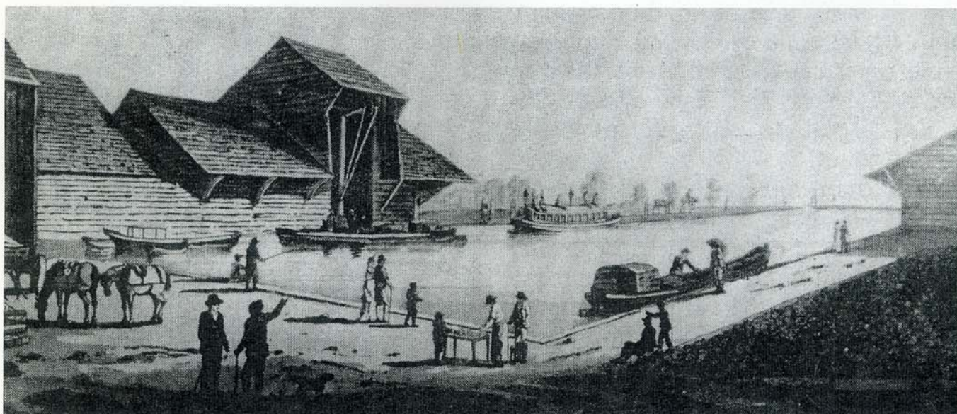
View at the head of the canal or basin at Paddington 1801. The boats from Hillingdon and West Drayton arrived at the end of the Grand Union Canal in horse drawn monkey barges and were unloaded under the unique umbrella roof (shown above)
